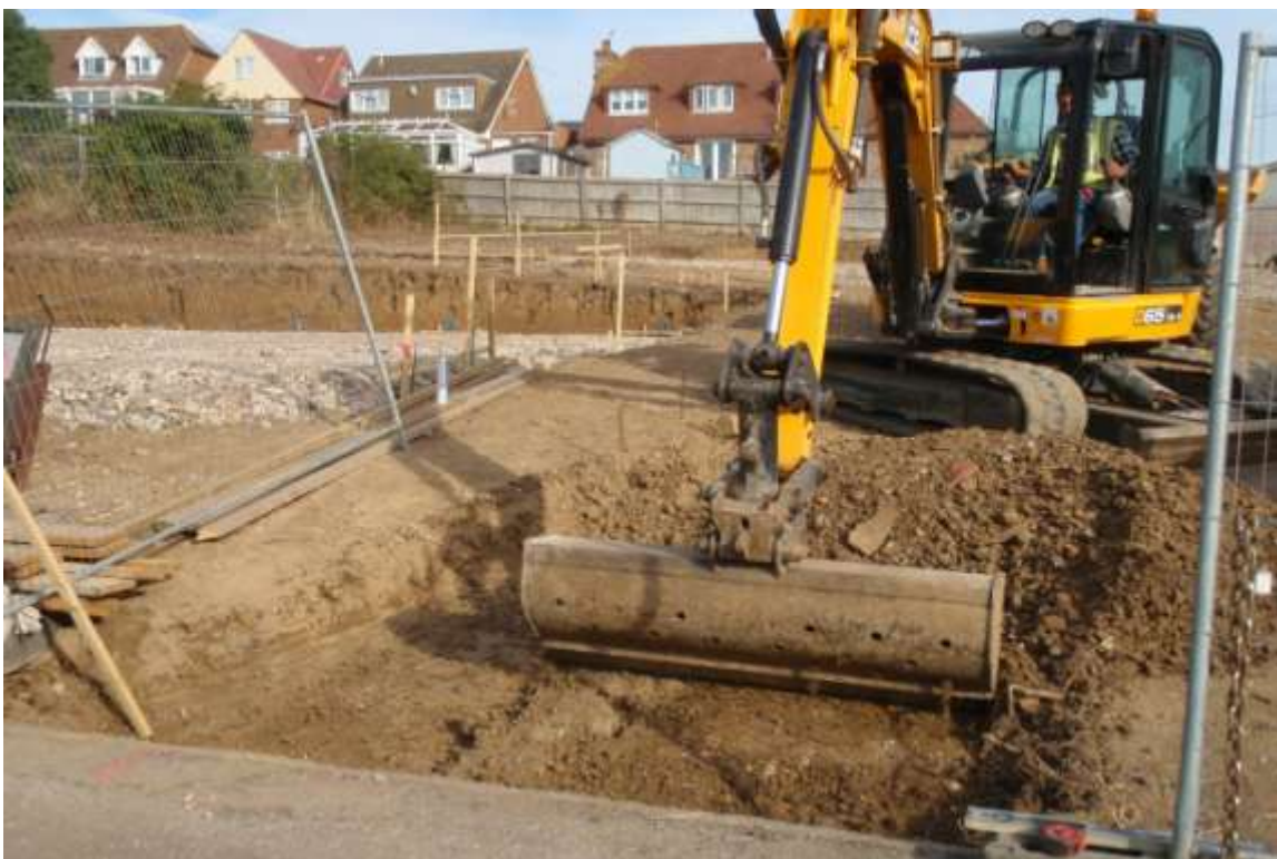
Plate 3. The site showing reduction of access road (looking north)
