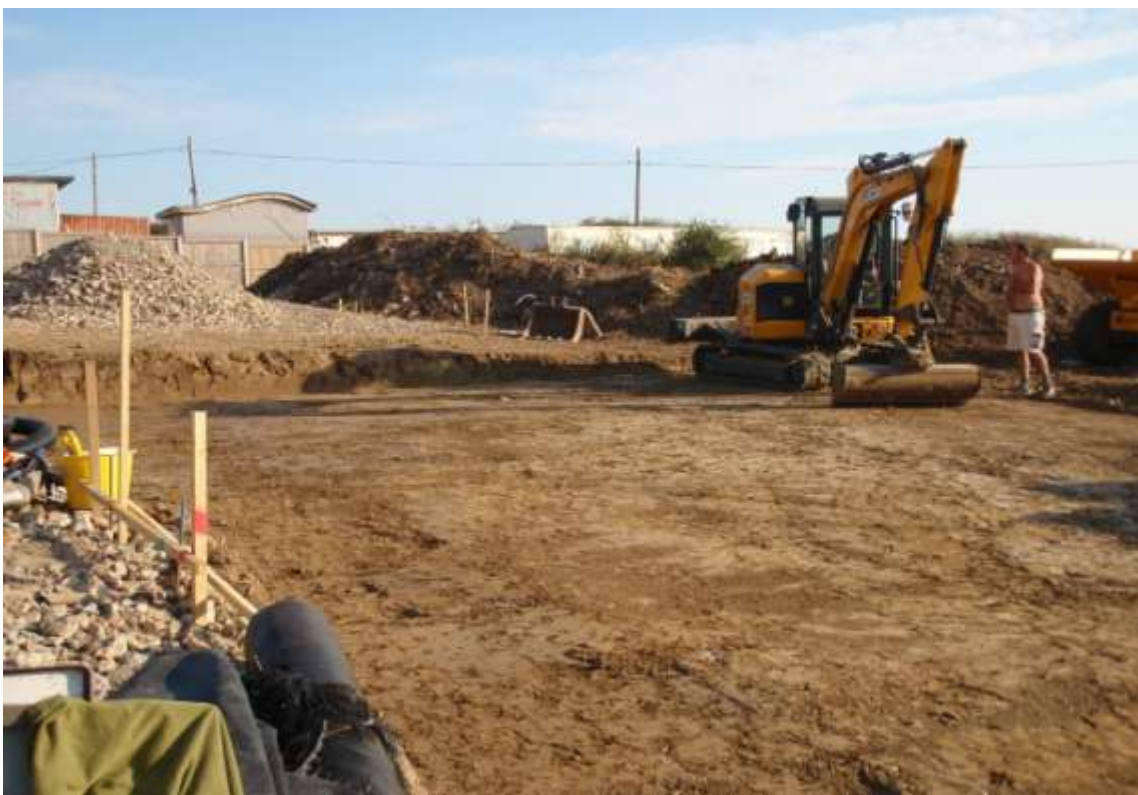
Plate 5. Reduction of site completed (looking north-east)
