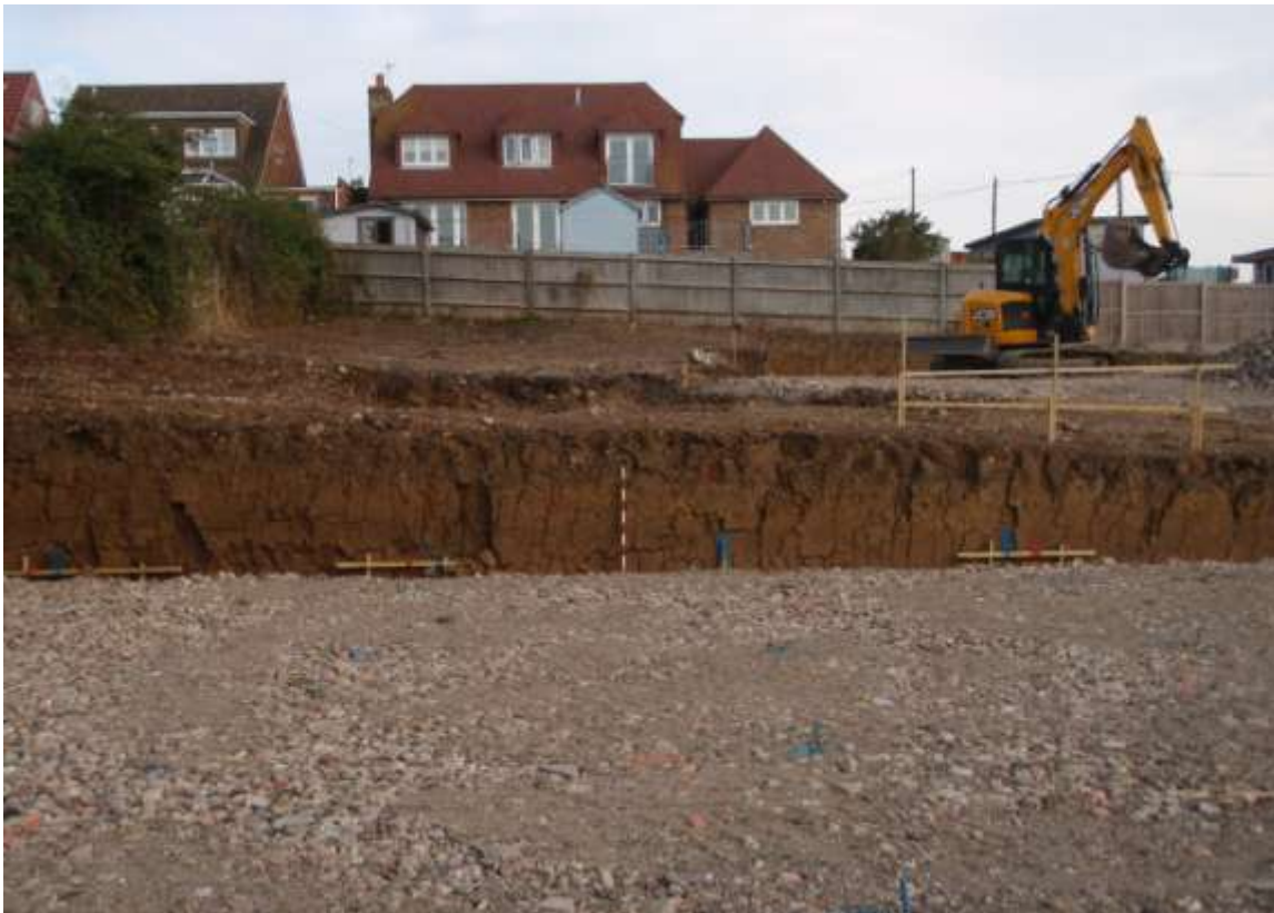
Plate 2. General view of site showing section through London Clay (looking north)
