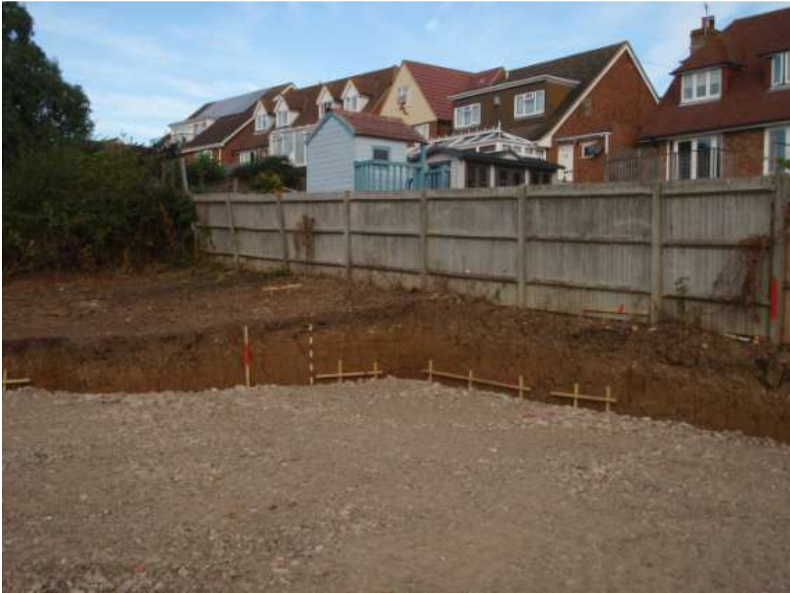
Plate 6. Inspection of vertical faces in Area 1
