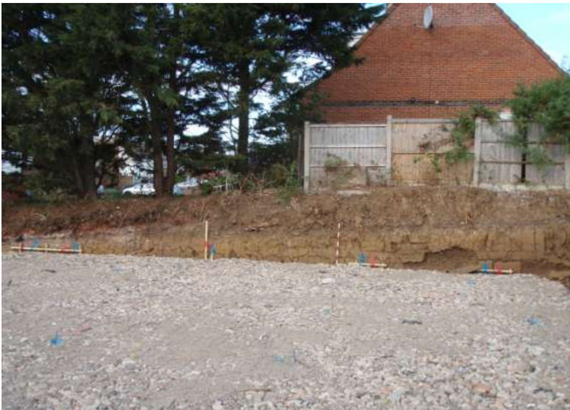
Plate 7. Inspection of vertical faces in Area 2.
