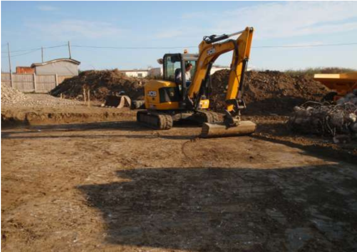
Plate 4. Reduction of site (looking north-east)
